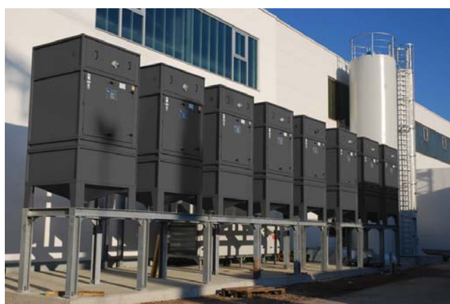
ZPF with adjacent fan in a soundproof housing
