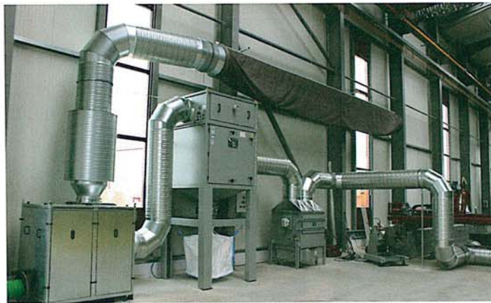
The extraction and filter unit "ZPF" takes in the polluted air and purifies it.
